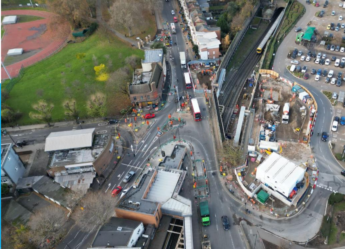
New Surrey Quays Station Ticket Hall, (January 2024)
