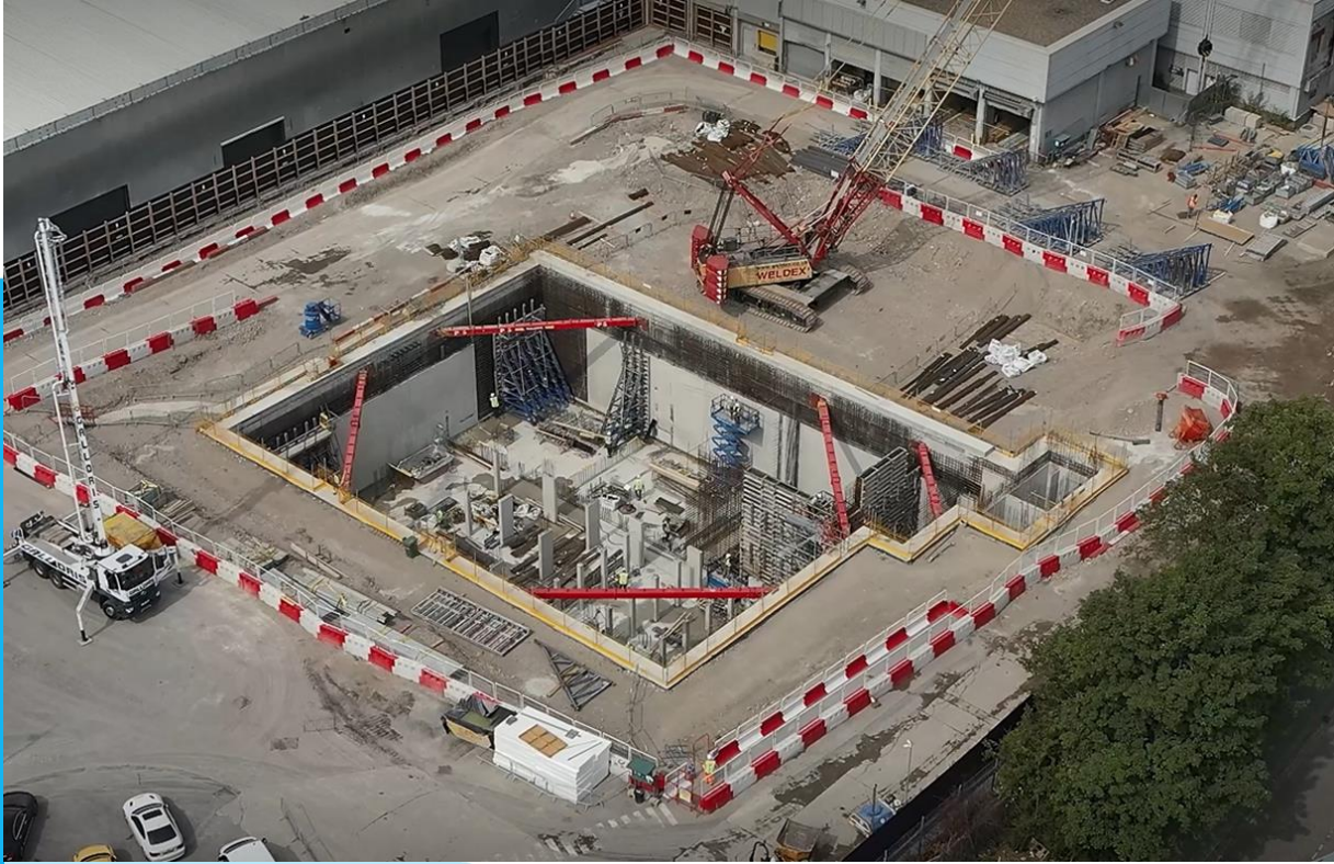
Sub Station under construction – early 2023 – Quebec Way
