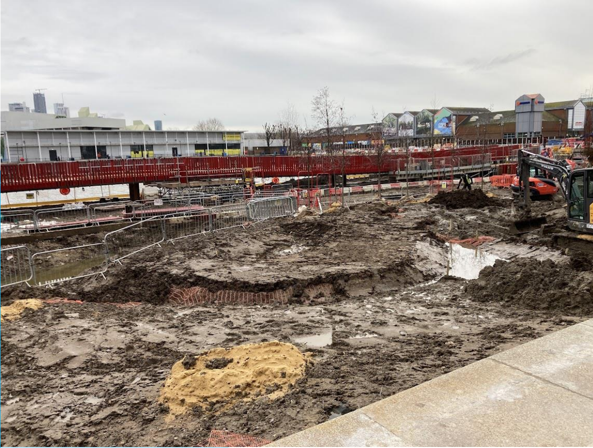
View from Deal Porters Way - relandscaping and tree planting, January 2024
