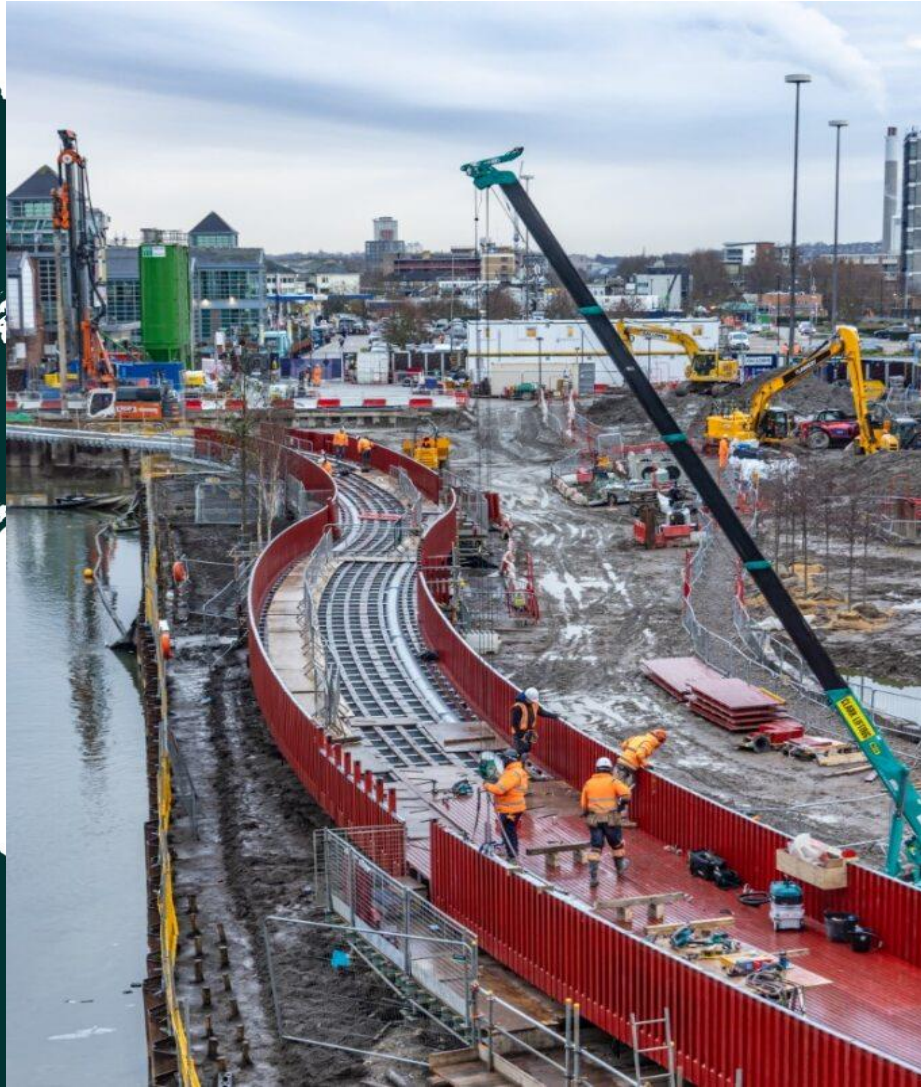
Boardwalk construction underway in Canada Dock (December 2023)
