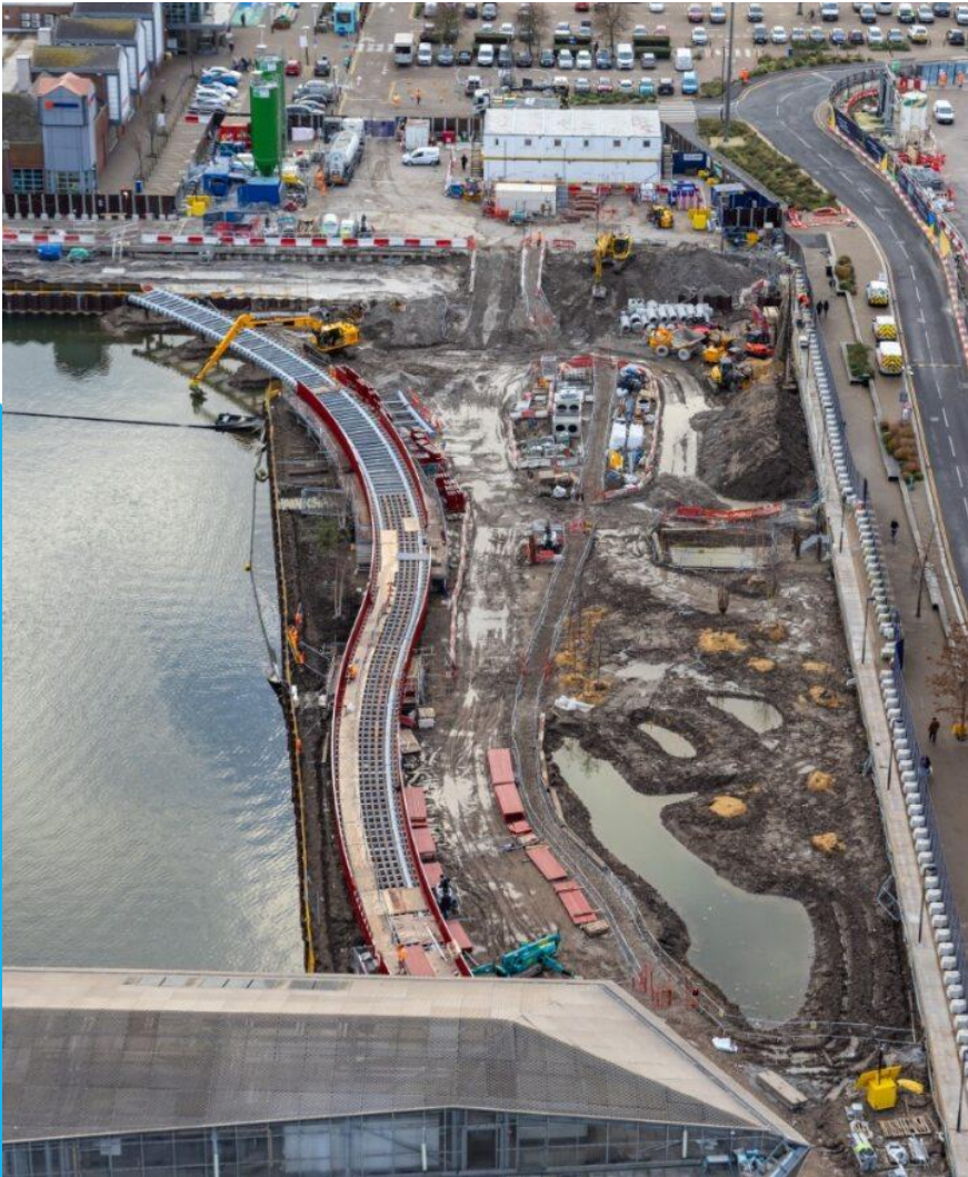
Aerial view of boardwalk construction in Canada Dock (December 2023)
