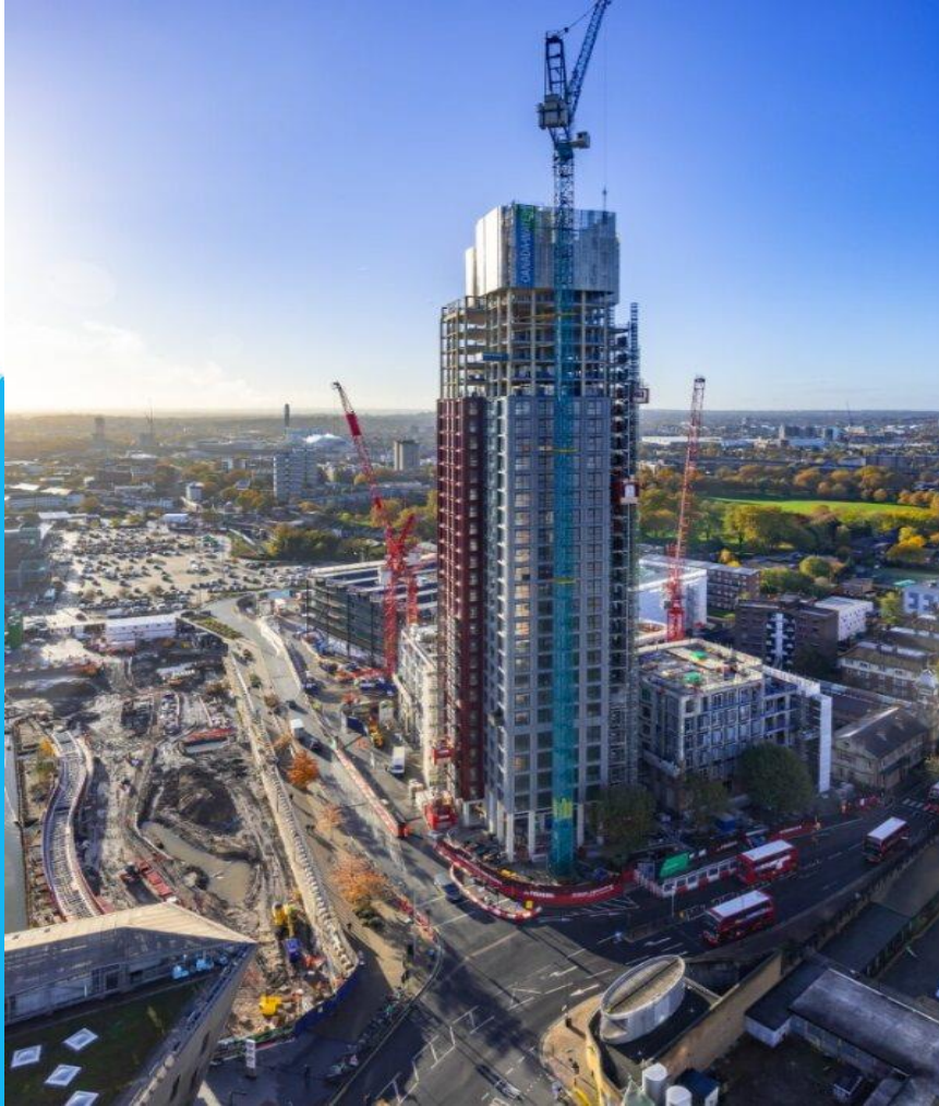
Construction of the façade of The Founding continues (December 2023)
