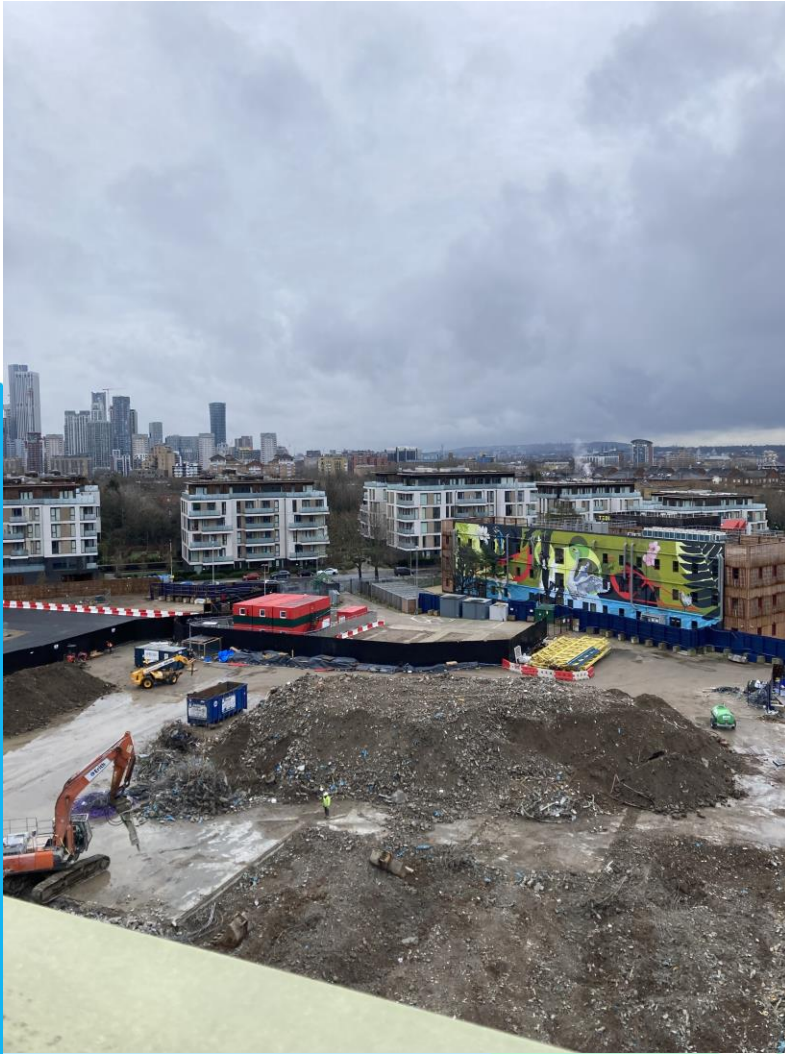
Aerial view of Printworks construction
