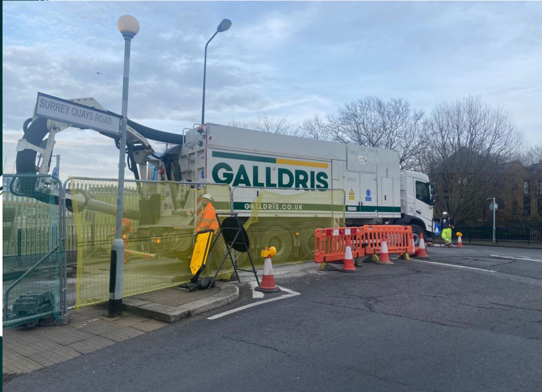
Works ongoing along Surrey Quays Road and Redriff Road
