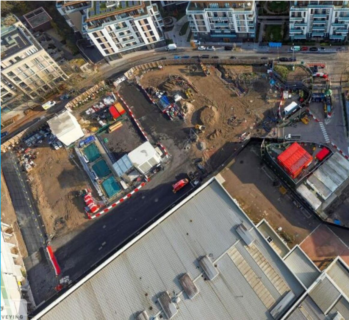
Aerial view of the below ground substation (December 2023)
