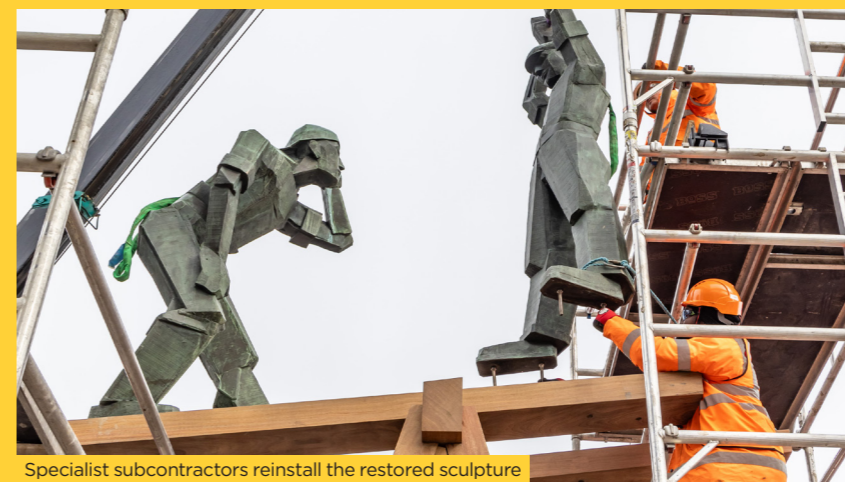
Specialist subcontractors reinstall the restored sculpture
