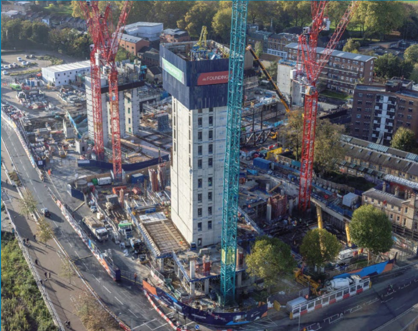
Pictured: Work being undertaken on Plot A1
