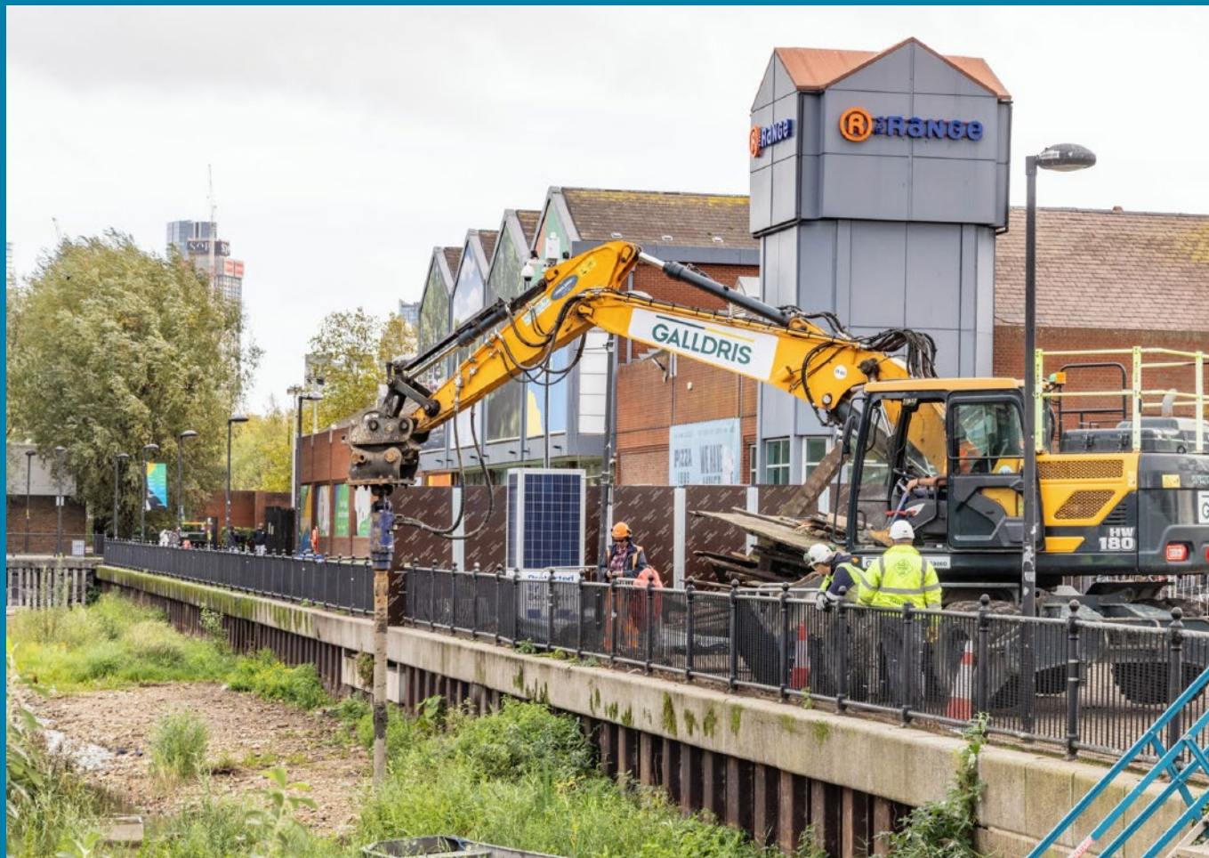
Pictured: Work being undertaken at the dock
