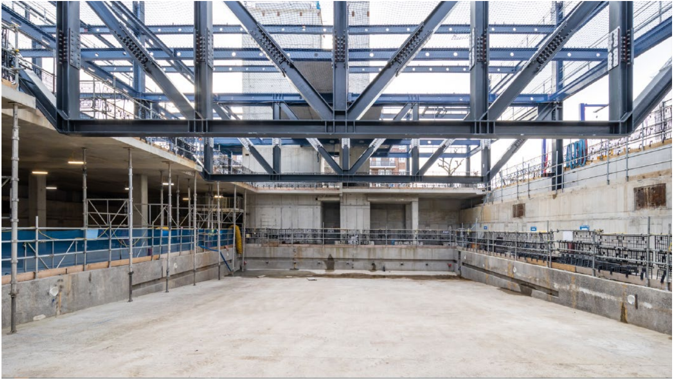
Pictured: Work being undertaken at Plot A2
