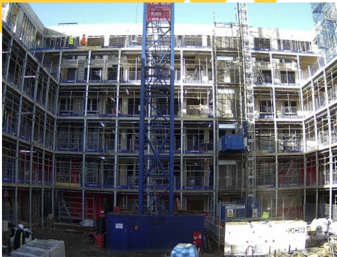
Pictured: Ongoing brickworks at Plot K1
