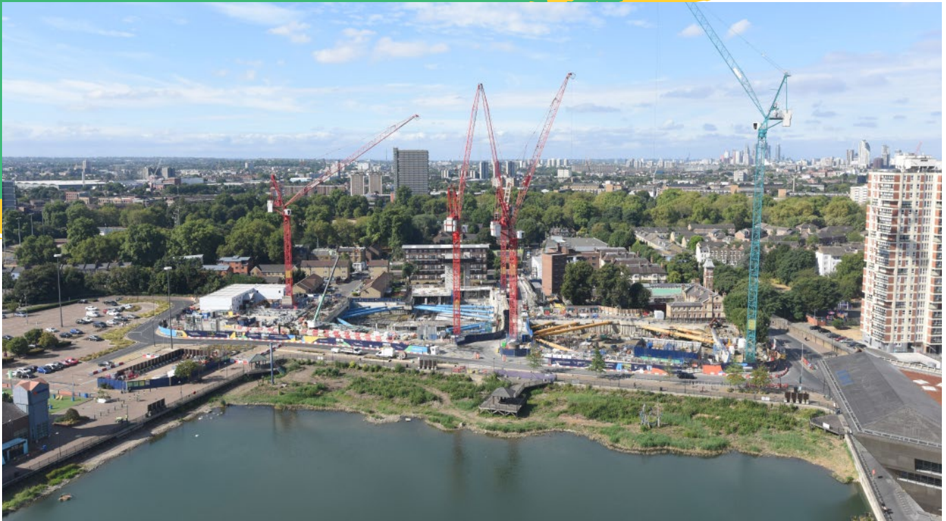
Pictured: View of Plots A1 and A2 from Canada Dock
