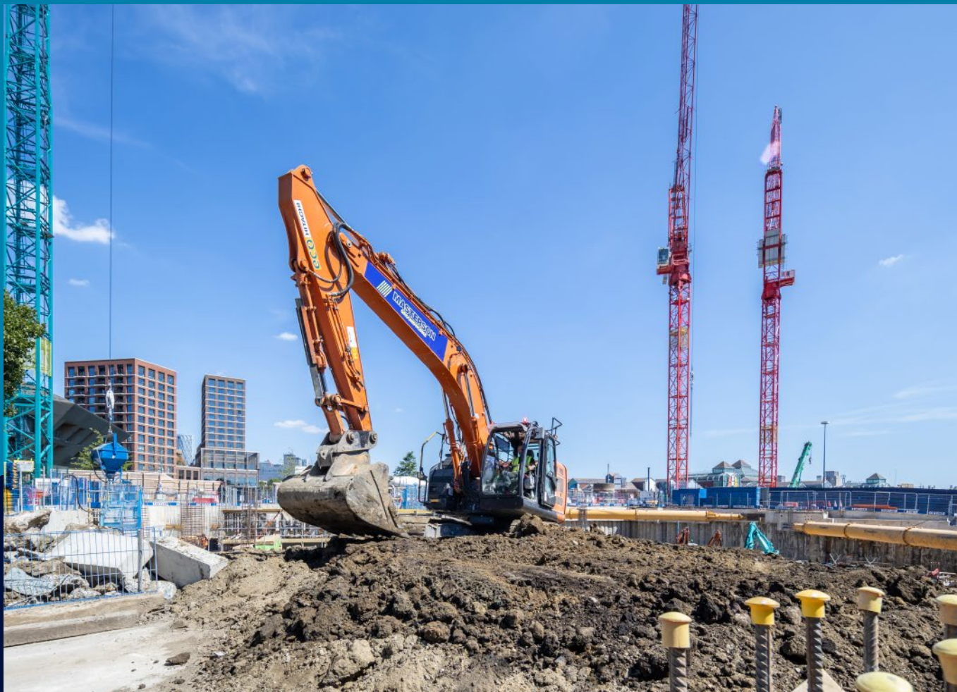
Pictured: work being undertaken on Plot A1
