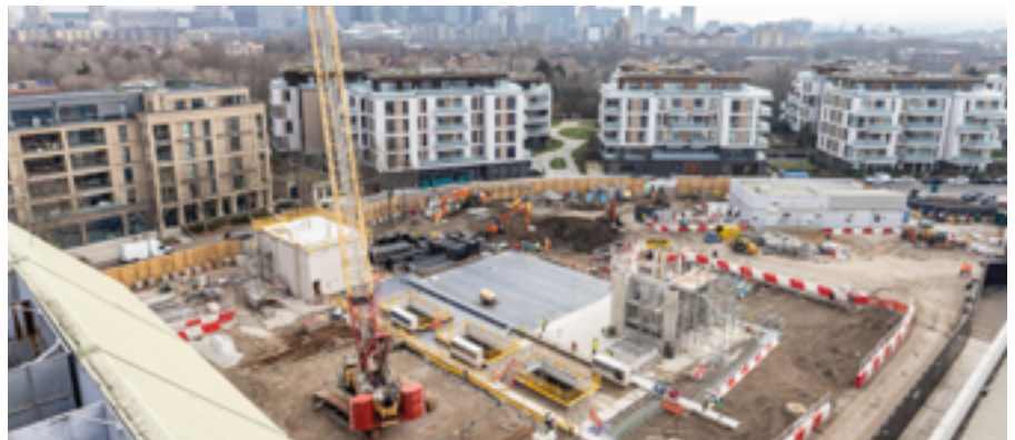
Pictured: Work being undertaken at the below ground substation
