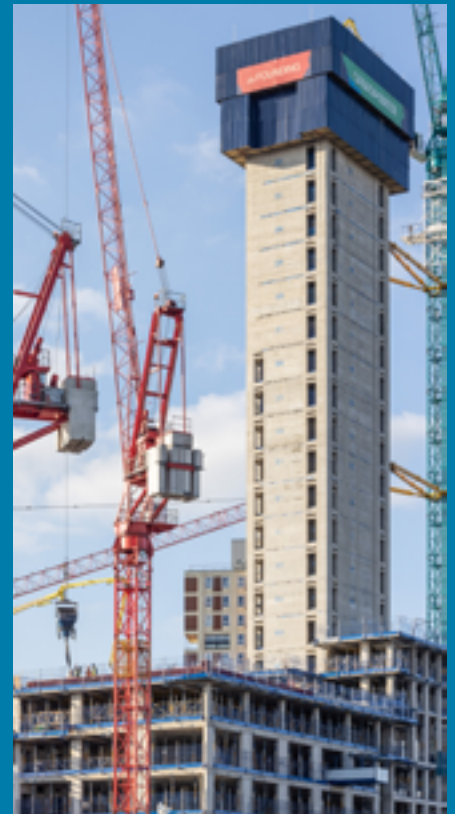
Pictured: Works being undertaken on Plot A1
