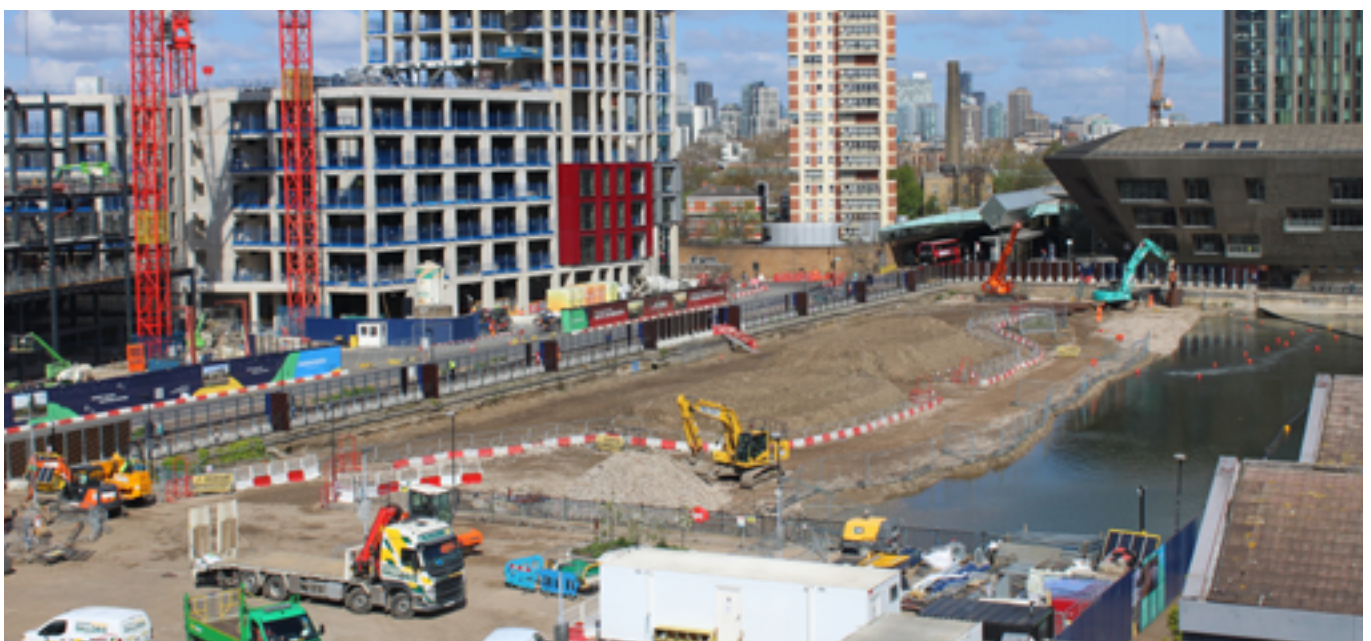
Pictured: Works underway in the dock
