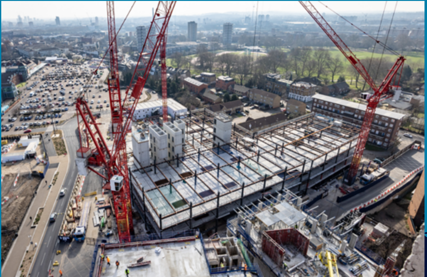
Pictured: Work being undertaken on Plot A2
