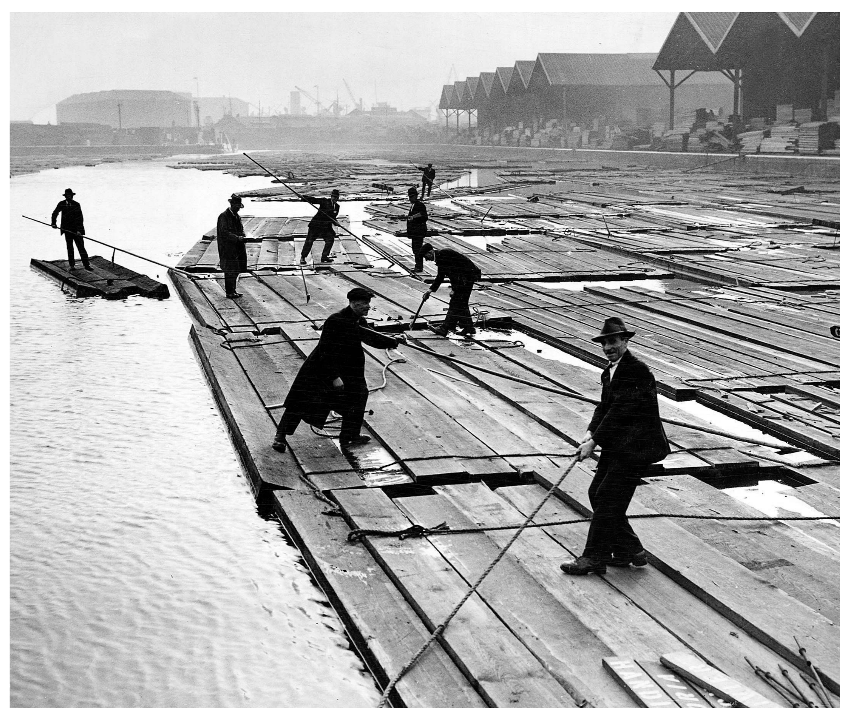
Reference images of the timber docks
